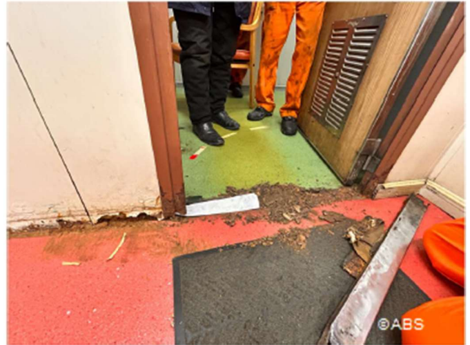
Crew mess room entrance door sill (Class-B fire door) and bulkhead panel wasted. Fire boundary integrity lost.
