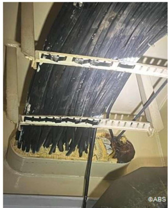
Multi-cable transit in the Engine Room workshop not as required – cable is run outside of the cable transit and improperly sealed.
